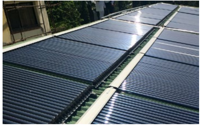
Sea Cliff Apartments - Dar es Salaam
